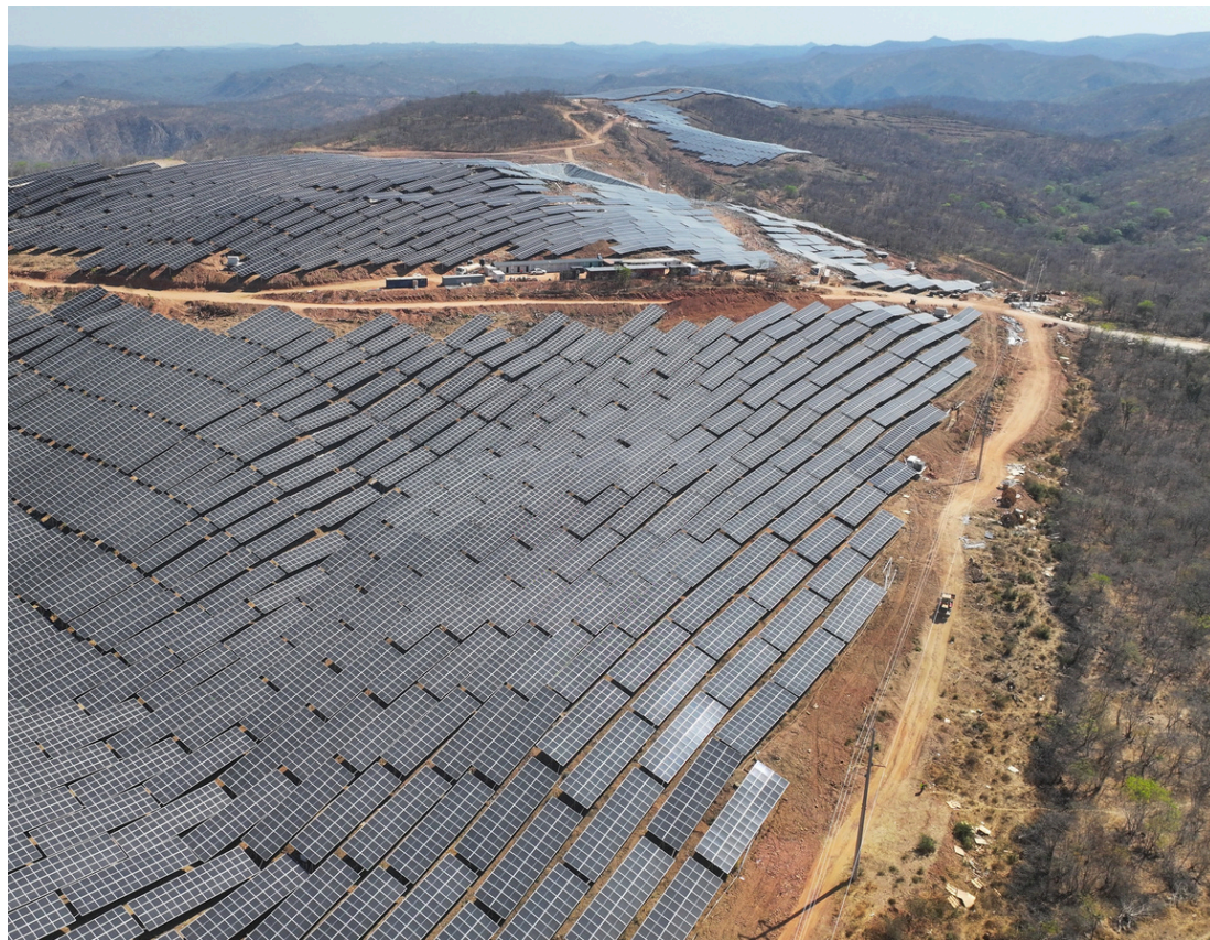
The Kamativi Solar Plant
